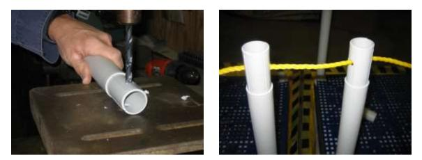
Hole was drilled at the top end of the poles that are to function as a railing; presents a flimsy but respected border along corridor so they don't jump off
