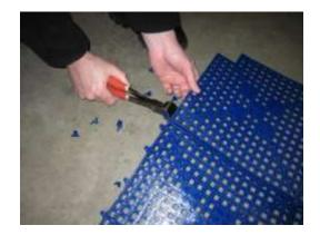
Six 12"x12" DriDek® panels were connected and their corners cut to accommodate the shelving poles. The edge connectors were trimmed to create a smooth edge.
