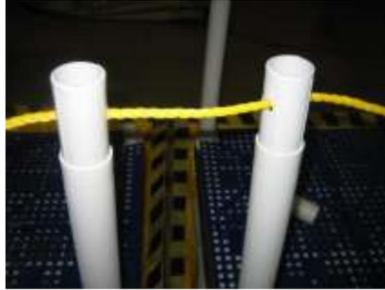
Hole was drilled at the top end of the poles that are to function as a railing; presents a flimsy but respected border along corridor so they don't jump off
