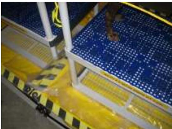
Assembled shelving units are placed within the two pools: one for the initial soap decontamination, next for water rinsing. A plastic sheet has been placed between the two pools to prevent contaminated water from falling through.
